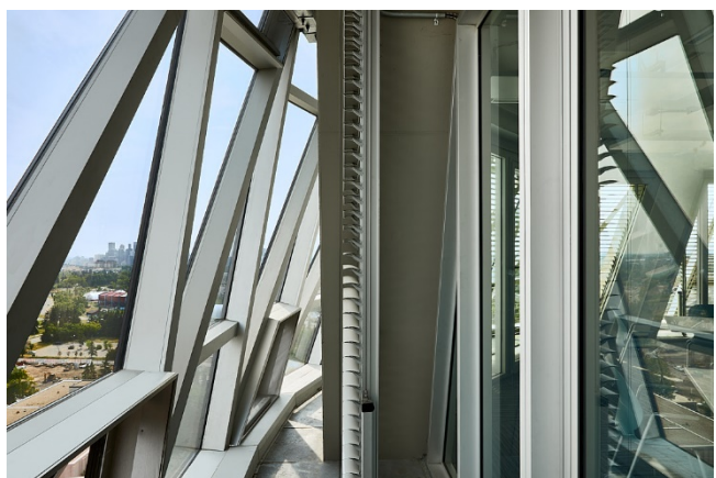
Figure 3: The active shading system within the double-skin facade and the building-integrated renewable energy generation contributed to the MacKimmie Tower's green building standard recognized by the Canadian Green Building Council (source: Hueck)
