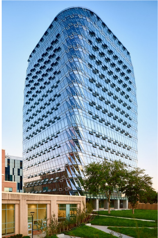
Figure 2: The MacKimmie Tower reawakens with a double-skinned 'breathing' façade that allows highly performant energy efficiency, continuous air ventilation and quality of interior lighting. (source: Hueck)
