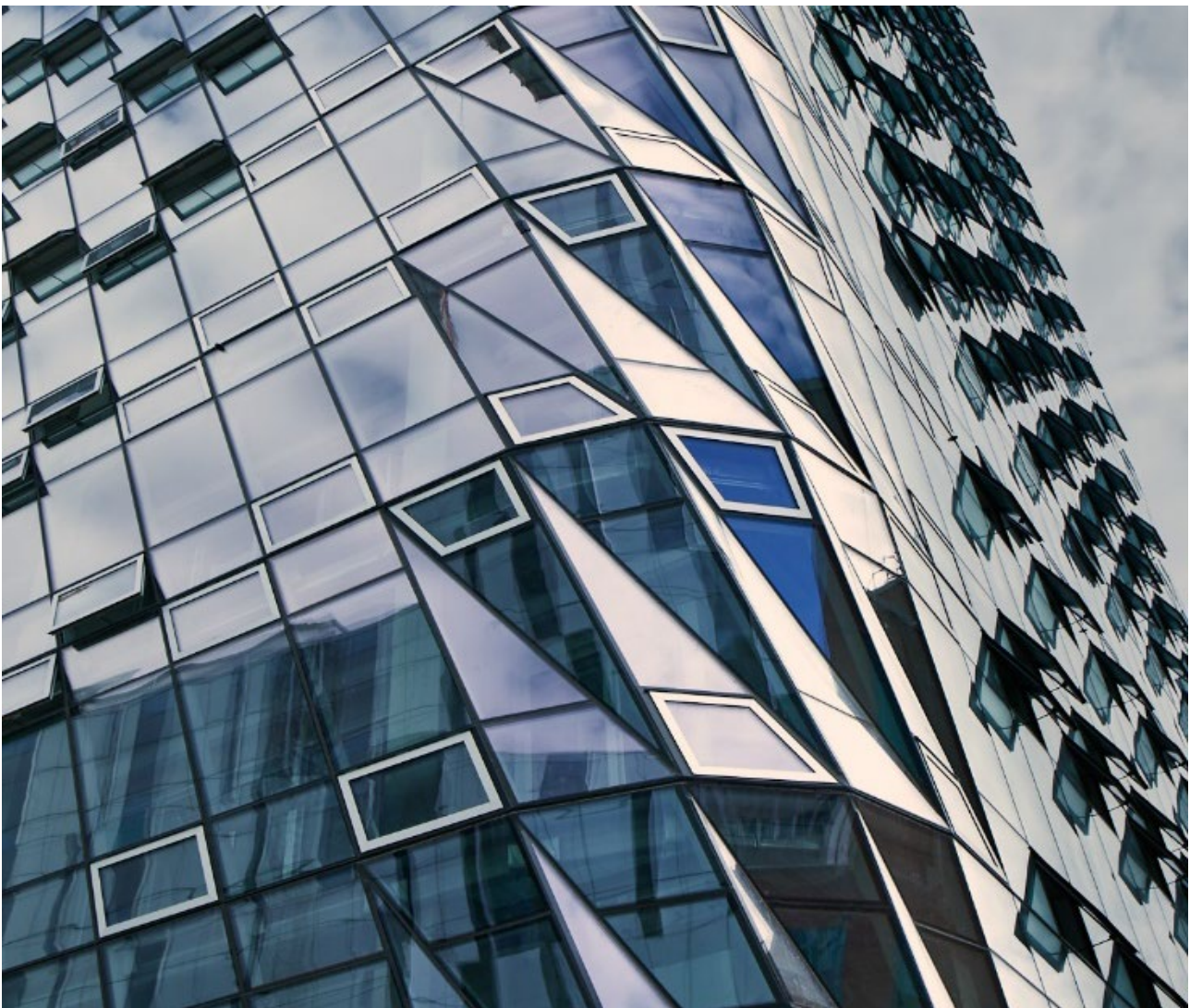
Figure 1: Concealed motors facilitate the automatic opening and closing of the windows, which are operated by the Building Management System, while retaining the harmonious look of the façade. (source: Hueck)
